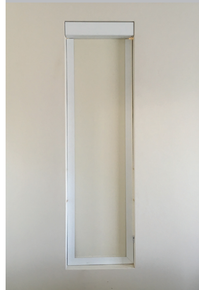
50mm channels used for room darkening
